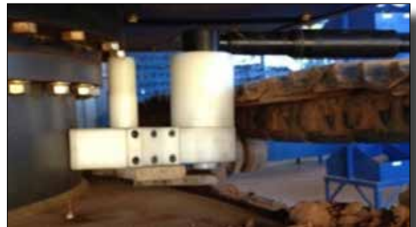
Final Assembly Tightening Car Swing Bearing
